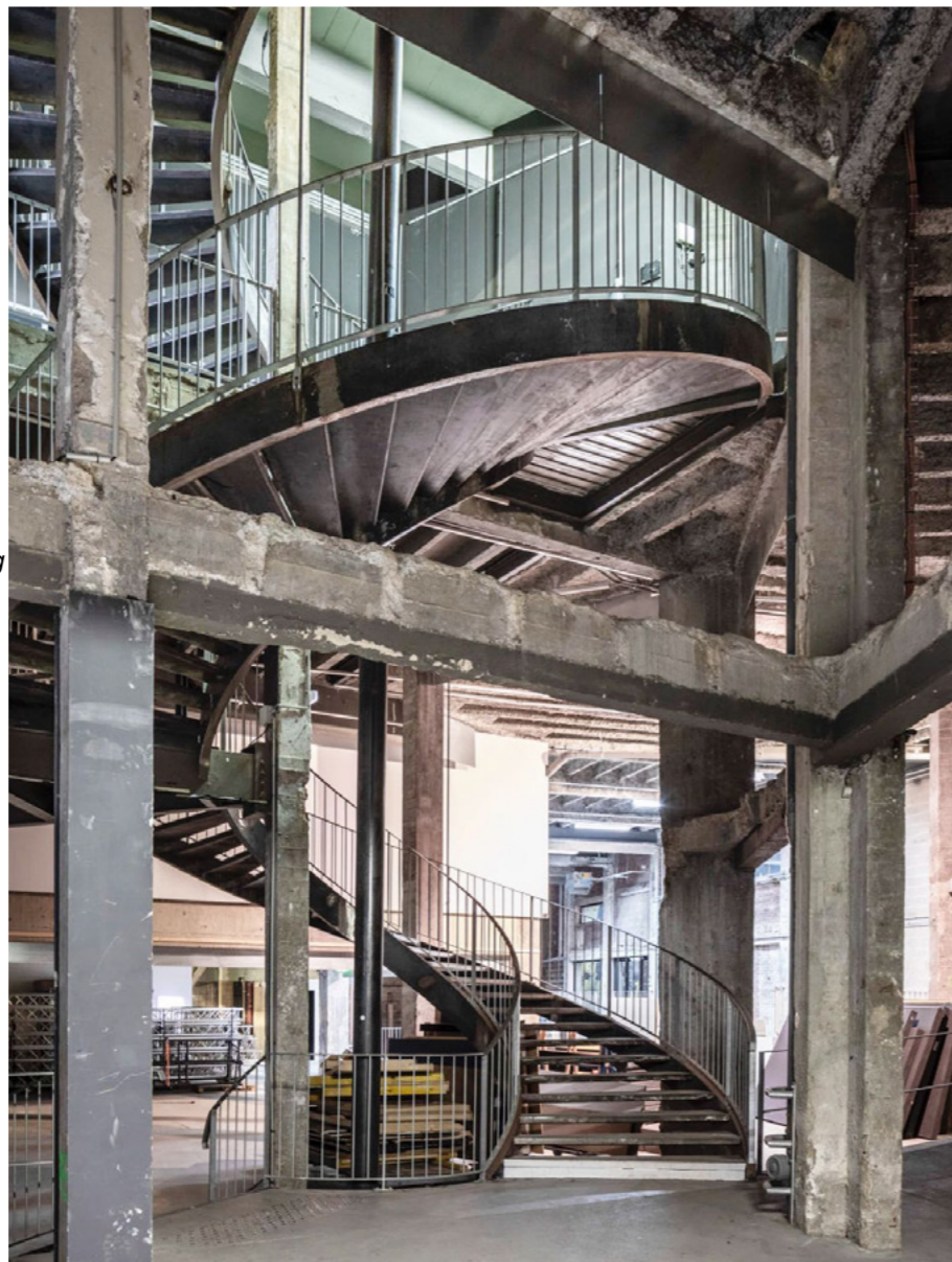
Right The Palais de Tokyo, Lacaton + Vassal, 2014. This renovation of the 1937 museum in Paris demonstrates a shifting of values in architectural thought-leadership. In this case, rather than being dismissed as unsightly, exposed concrete structure is celebrated for its ongoing functionality and augmented with modern additions.
