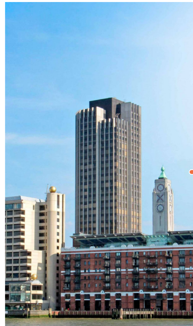
King's Reach Tower, Stamford Street, Southwark
